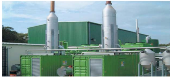
Holsworthy Biogas, Devon (2696 kW)
