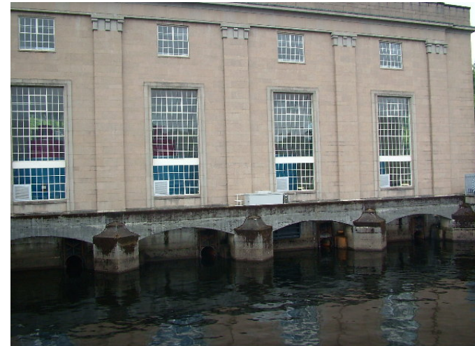
The tailrace pool into which water from the turbines is discharged.
