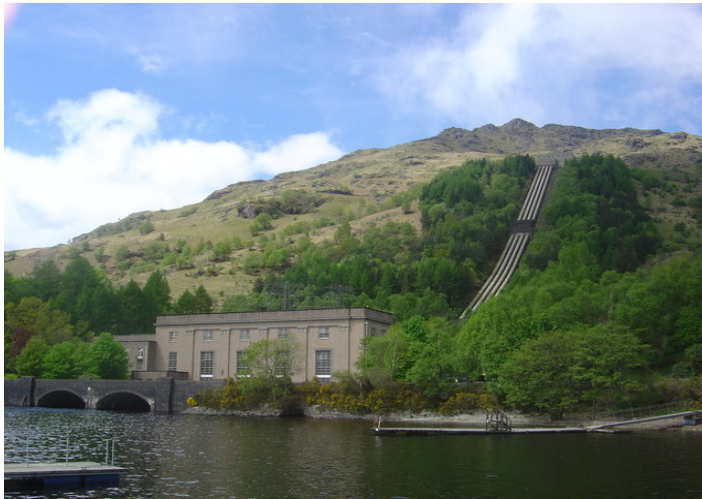
Four cast iron pipelines convey water down the steep hillside to the turbines.
