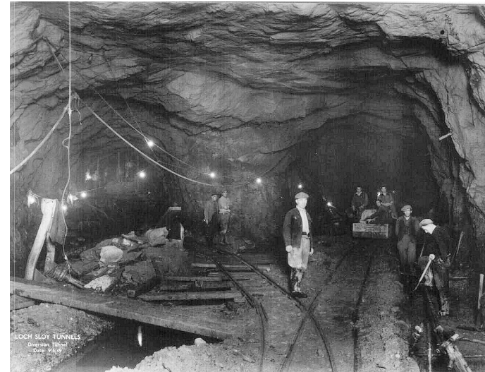
Sloy Power Station (> 20MW)
