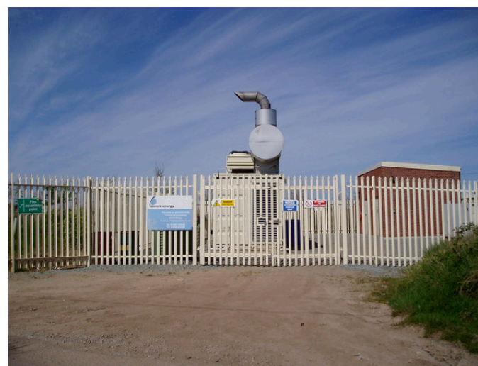
Generator at landfill south of Wangford 2
