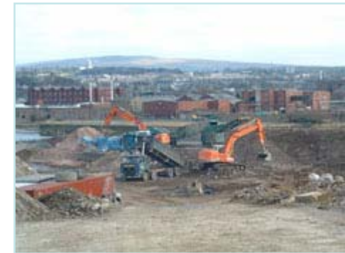
Salt Ayre Power, Lancaster (1136 kW)
